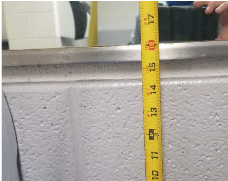
As Built: The mirror is mounted at 52" AFF which is too high.
