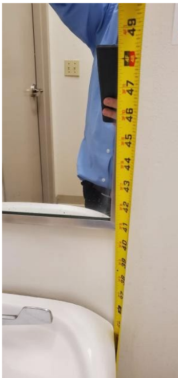
As Built: The mirror is mounted too high.
